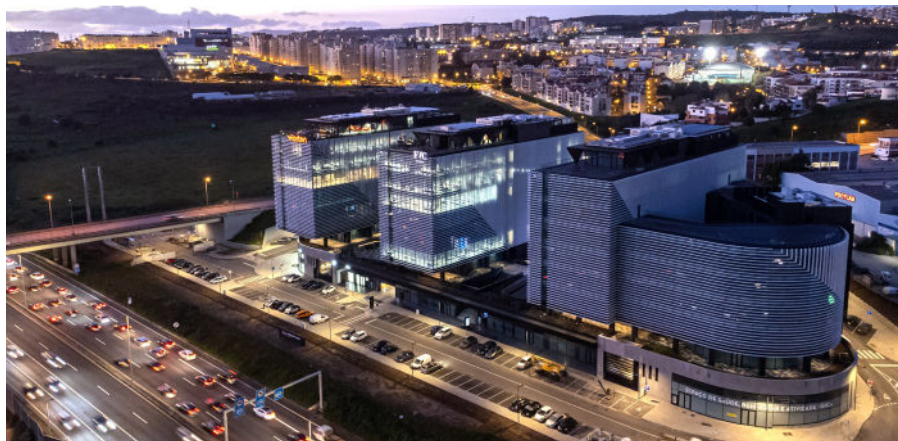
Exemplary energy efficiency and tenant friendliness combined in the new Lisbon World Trade Center.
